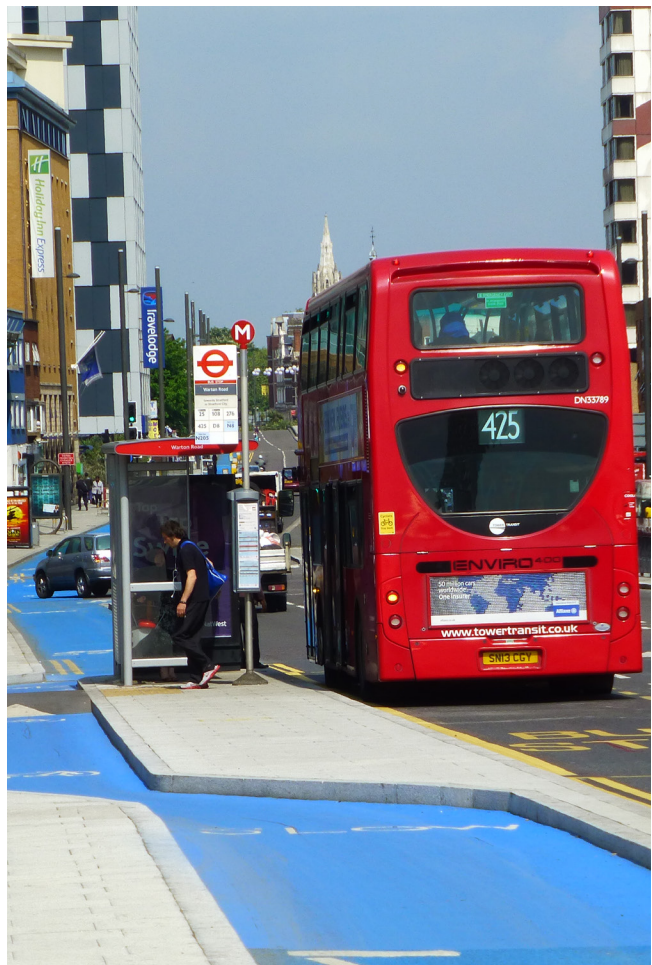
Cycle Superhighway2 and an island bus stop which avoids conflict between cyclists and buses which stop here - Stratford High Street, London. © spsmiler
